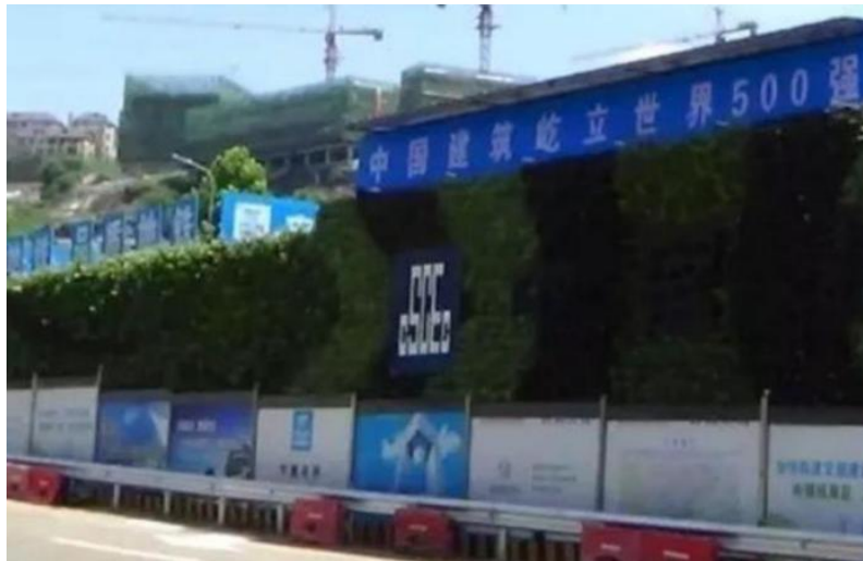
Fig. 11 The real scene of the green plant background wall of the 12th section of Chongqing Metro Line 9
