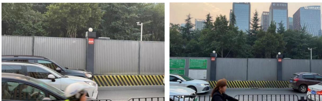
Fig. 1 Site Map of Xi'an Metro Construction Project
